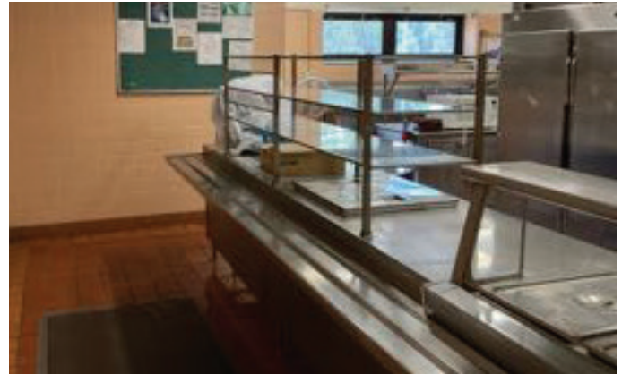
Wheeler Elementary: Existing serving line is 50+ years old with no way to modify or replace parts. Inefficient flow.
