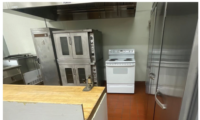
Rockwell Elementary: Double deck convection oven is very old and beyond its useful life. Bottom oven does not work, forcing staff to use residential range for warming.
