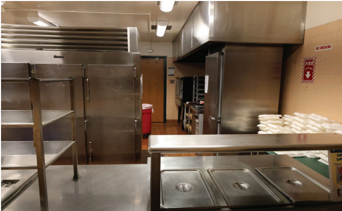
Wheeler Elementary: Exhaust hoods are beyond their useful life and need replacement.
