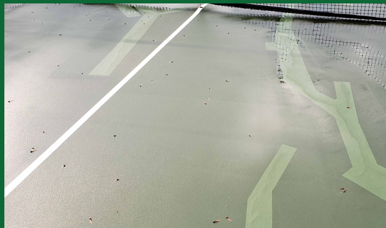
Tennis Court Resurfacing
