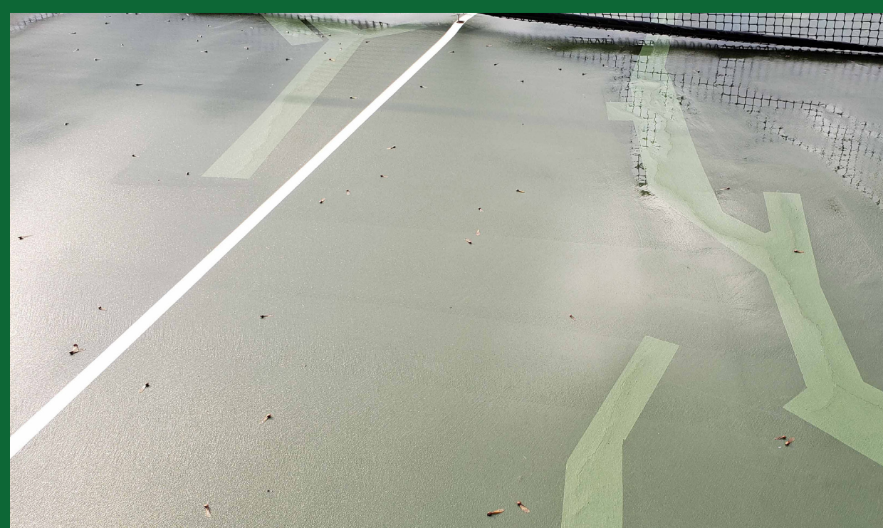
Tennis Court Resurfacing
